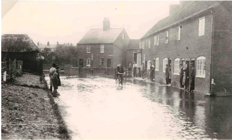
Floods in School Road, Alcester c1950 (ADLHS Collection)
